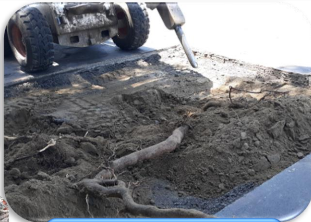
The asphalt has been removed and one of the roots that caused the problem is being cut away
